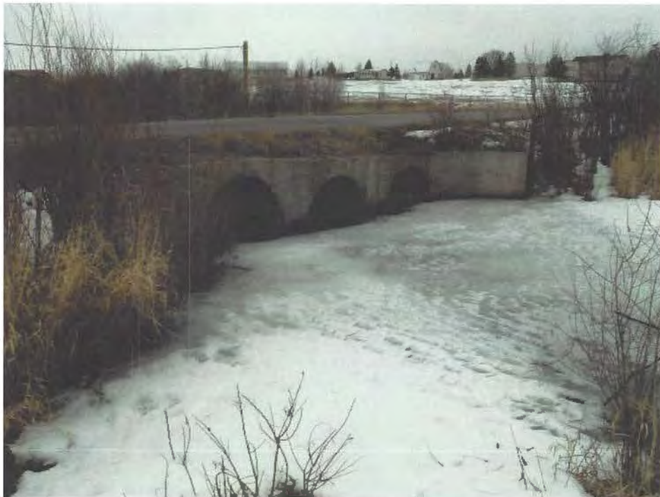
ELEVATION LOOKING NORTHEAST
