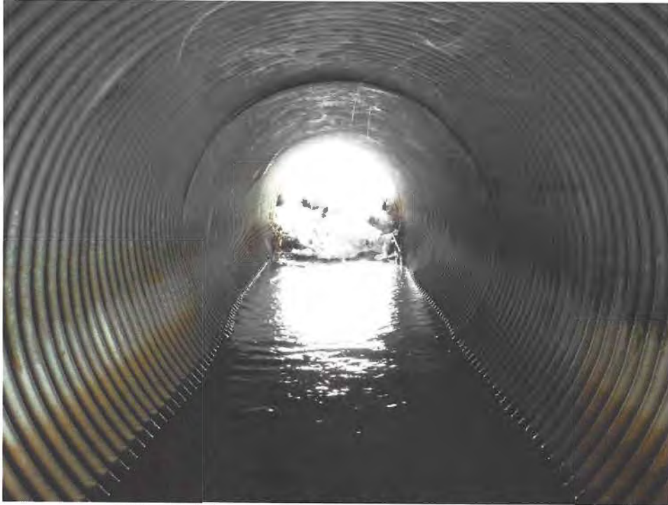
UNDERSIDE VIEW LOOKING SOUTH, PIPE 3
