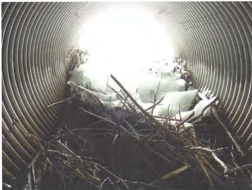
DEBRIS AND ICE AT INLET OF PIPE 2
