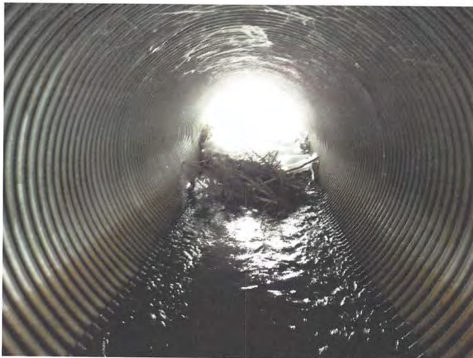
UNDERSIDE VIEW LOOKING SOUTH, PIPE 2
