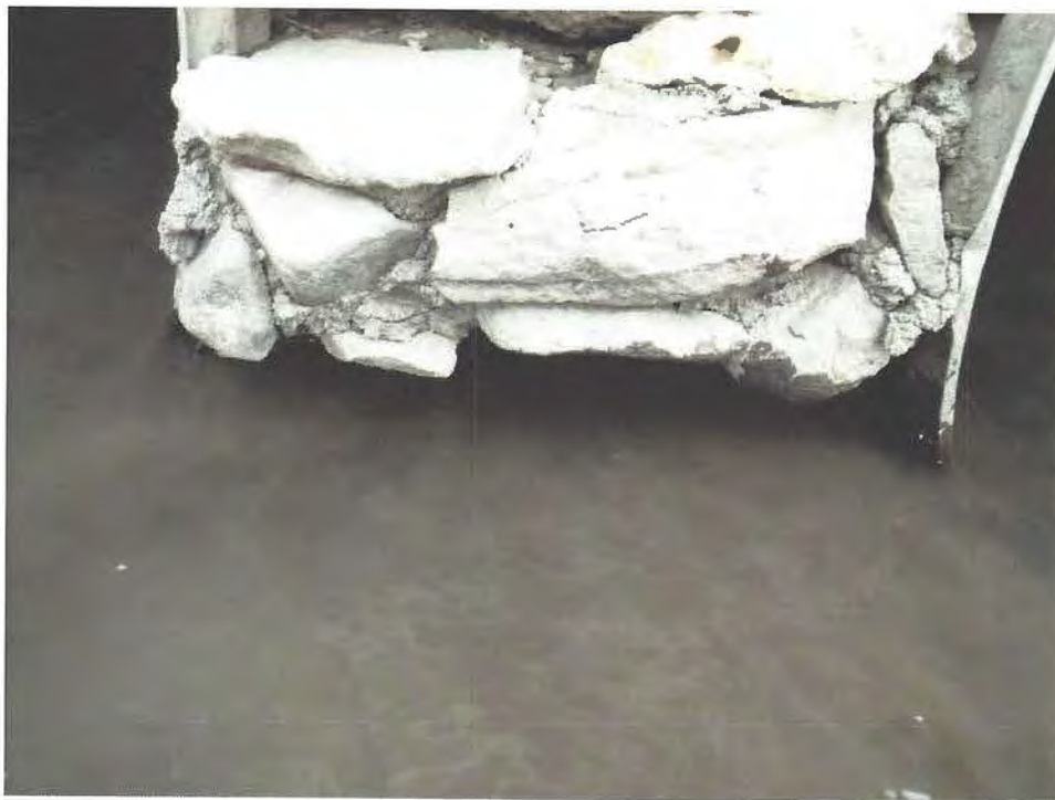
UNDERCUTTING OF PIER 3, DOWNSTREAM SIDE
