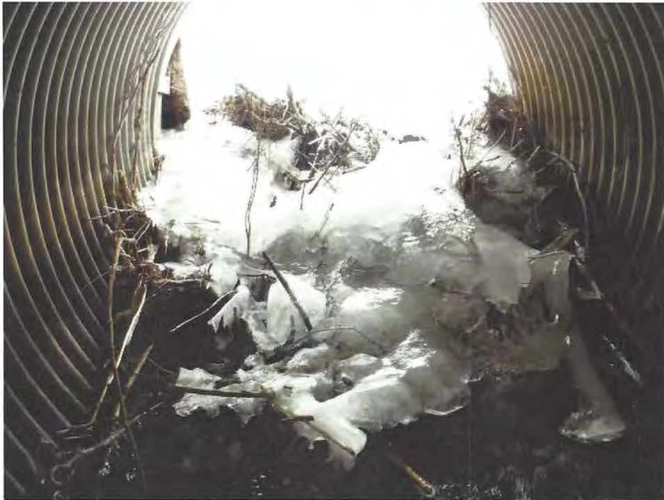
DEBRIS AND ICE AT INLET OF PIPE 3
