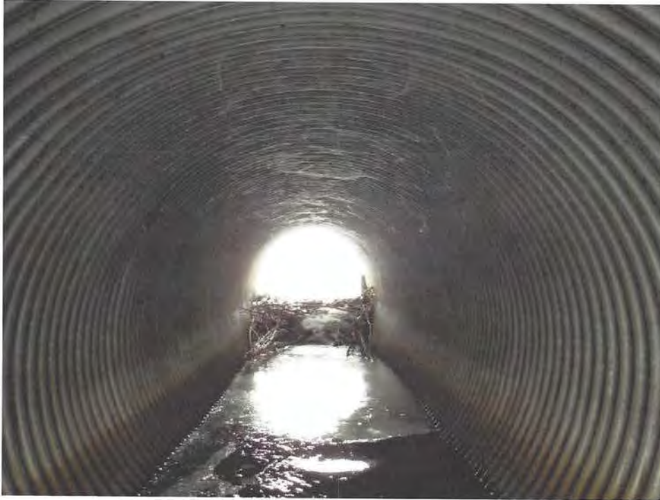
UNDERSIDE VIEW LOOKING SOUTH, PIPE 1
