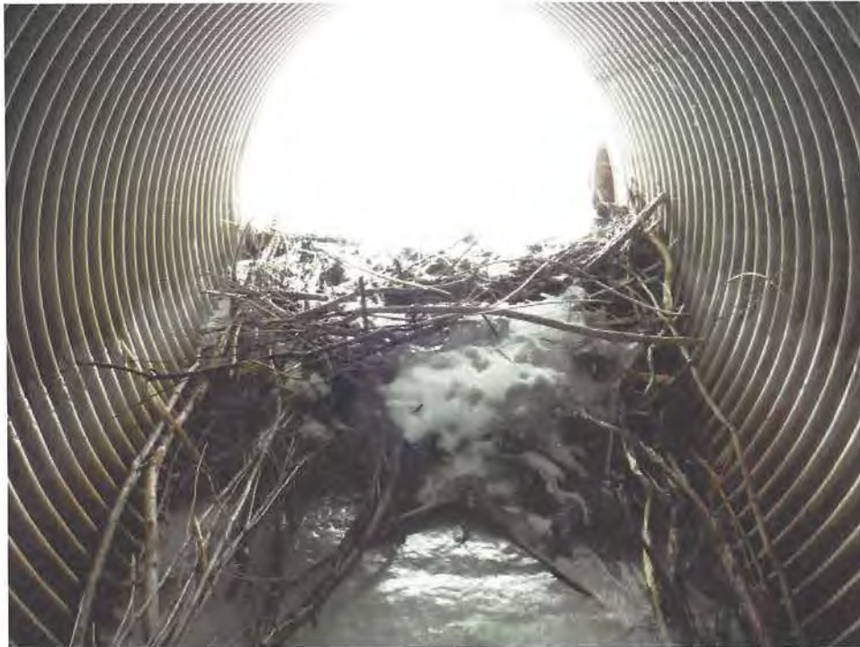
DEBRIS AND ICE AT INLET OF PIPE 1
